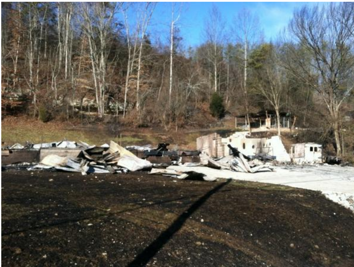
Figure 13 - House destroyed Sissonville, West Virginia . This house is one not replaced as shown in Figure 8.
