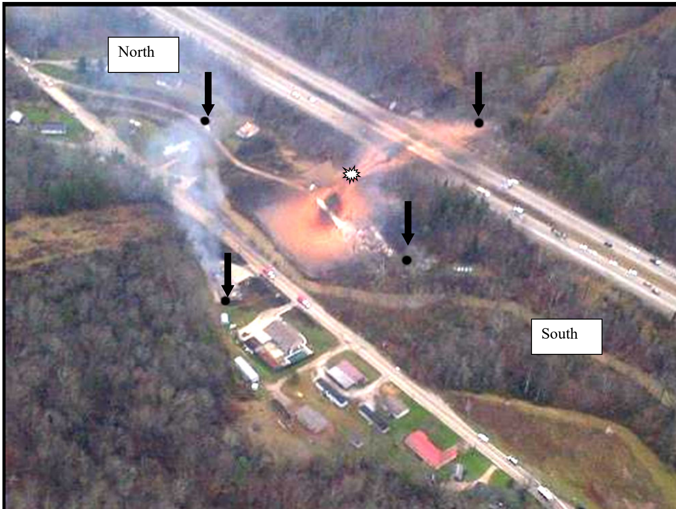
Figure 9- Aerial View showing approximate Locations of Heat Damage, Sissonville, West Virginia. Note the smoldering house to the west of the point rupture. This house was not replaced nor was the adjacent house to the south. See figure 8
