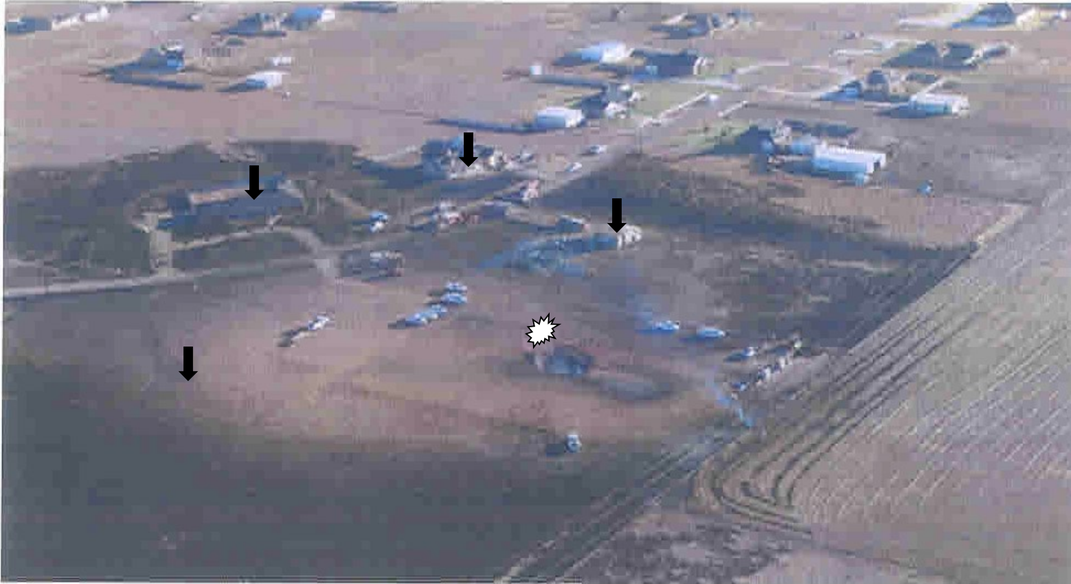
Figure 1- Pipe Rupture 11/5/2009 Bushland Texas Ref 12
