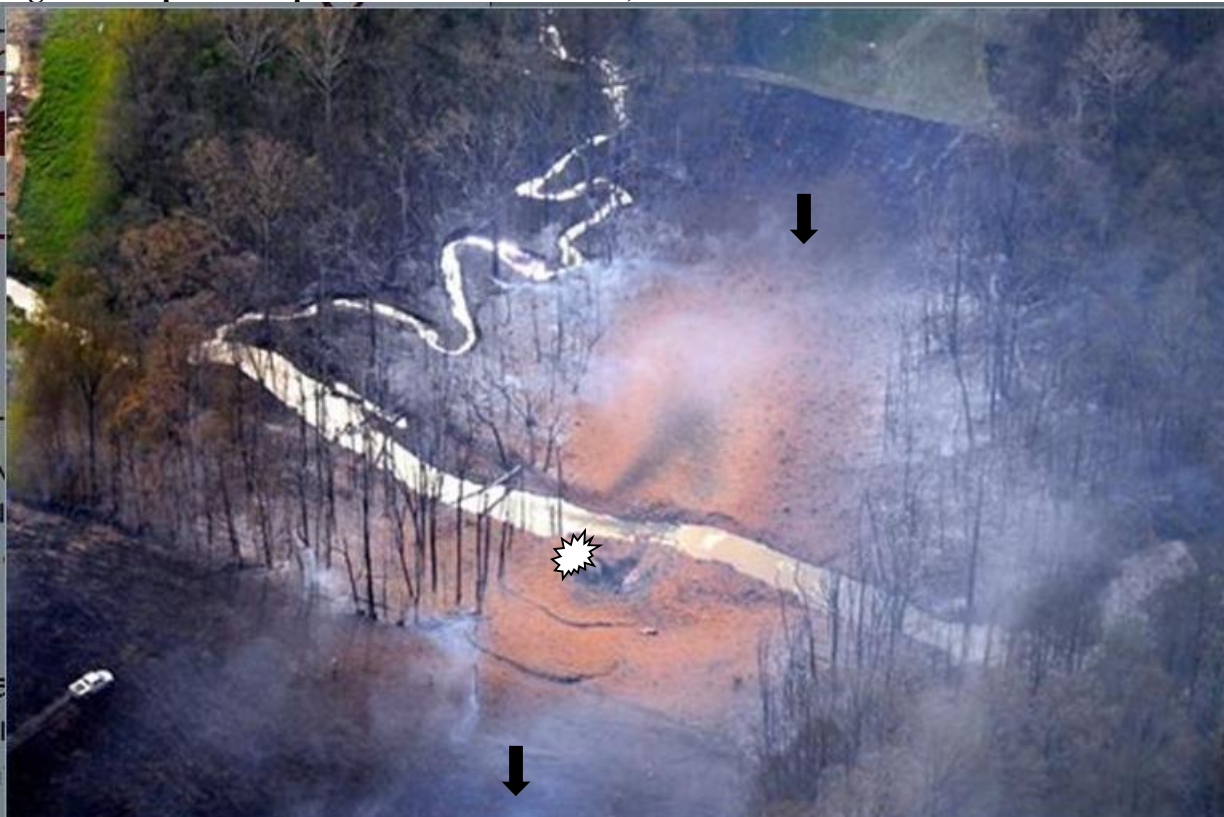
Figure 4- Pipeline Rupture 5/5/2009 Rockville, In Ref 16
