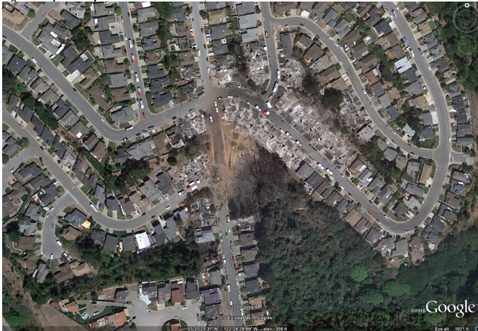
Figure 7- Pipeline Rupture 9/9/2010 San Bruno, Ca Ref 13
