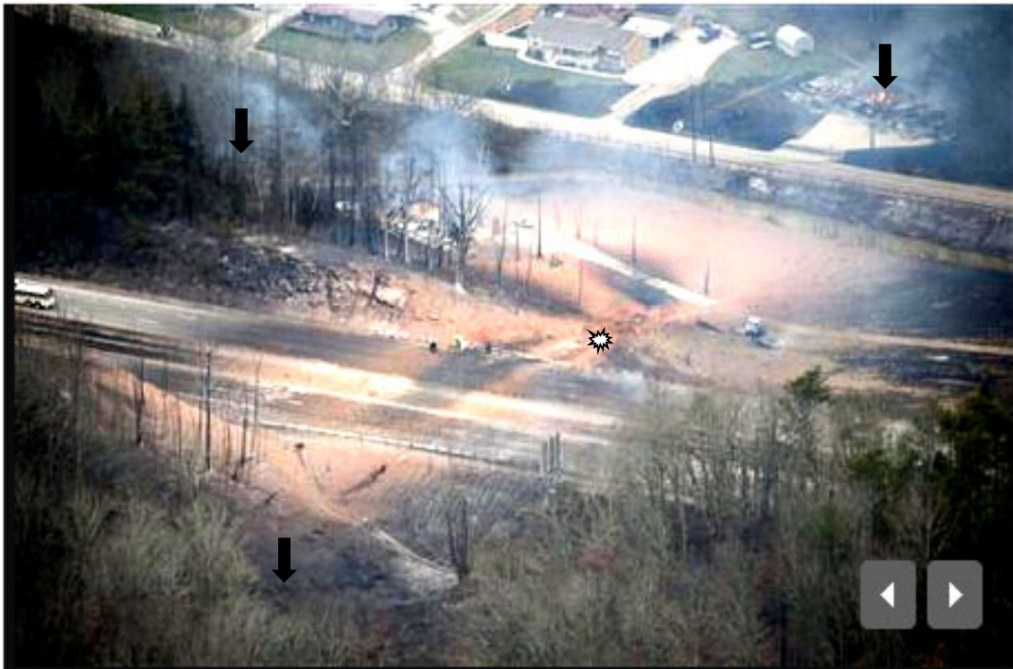
Looking From the East toward the West, Sissonville, West Virginia. Note the large areas of baked soil and scorched I-77.
