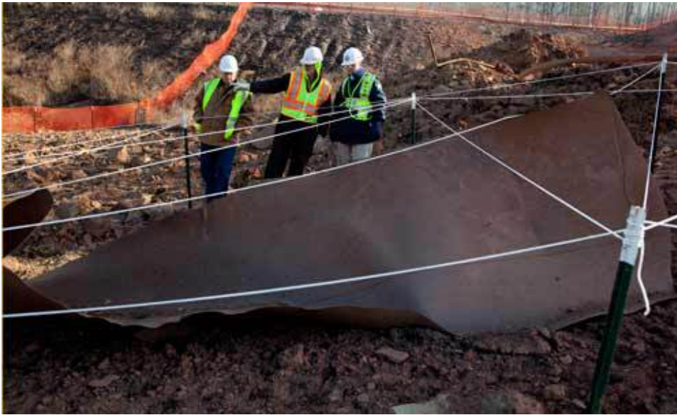
Figure 12- Pipe projectile Sissonville, West Virginia. Located 40 feet from the point of pipeline rupture.
